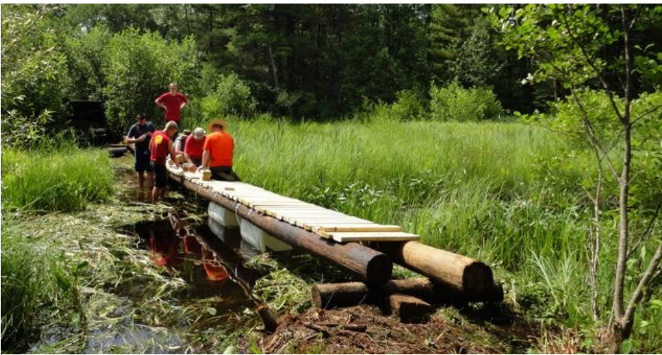
The boardwalk under construction.
