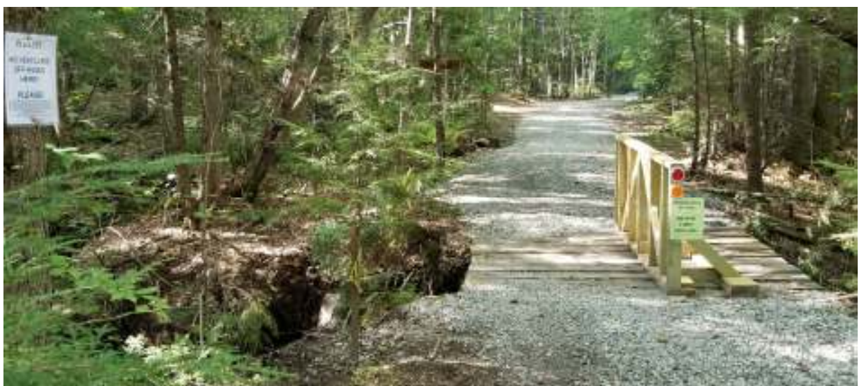
The road and bridge after improvements. Dan Hester built the removable railing to reduce the damage to the bridge. The distant part of the road is where the big mud hole had been, and the muddy water used to drain down the road almost to the bridge.
