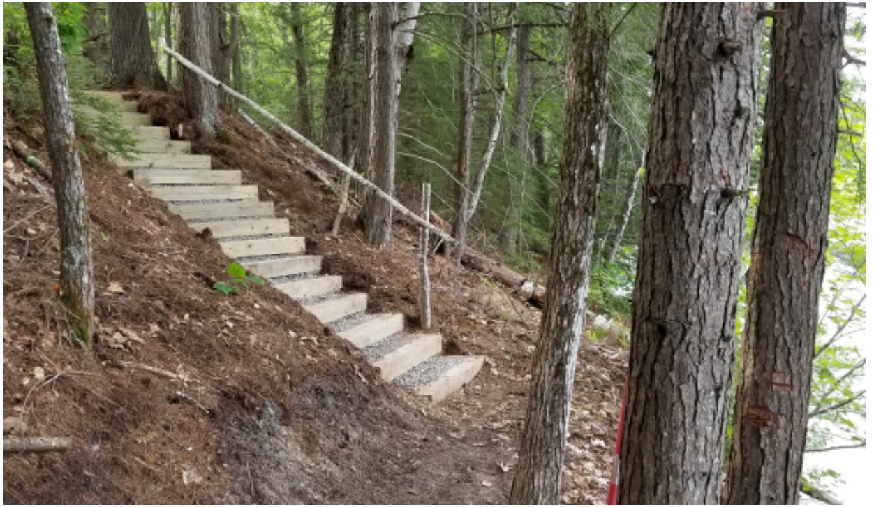
Karl Gifford of Sebago Stonework built a stairway of infiltration steps to descend from the higher level of the road down to a natural shelf closer to the normal river water level. During a spring high water, these steps will be partially submerged, and at a time of major flood they will disappear under water. However, we expect these to resist erosion damage and to remain usable for many years.
