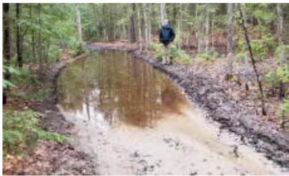
Improving the River Road has had its challenges. This photo shows the largest of several mud holes in the road on April 30 of 2020. Heavy vehicles and poor drainage had made it nearly impassable.
